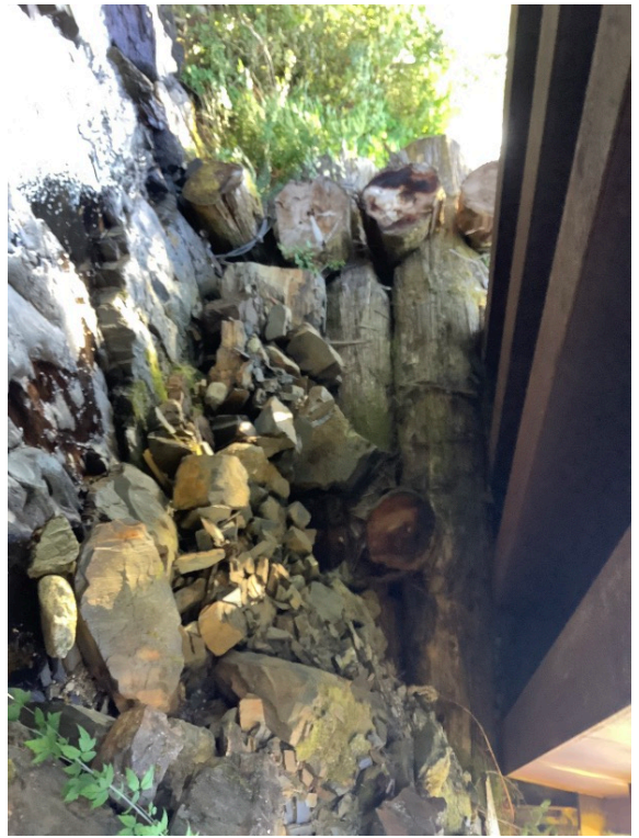
Right Bank Abutment when facing downstream
